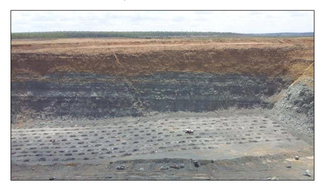
It was decided to pour (Auger) WALA heavy blend (60/40) into dewatered blast holes immediately after de-watering is conducted. The MPU and the de-watering truck where following each other in two separate rows to minimise the return time for the return of dynamic water back in to the blast hole. The blast holes where 270mm in diameter and average 30meters deep.
